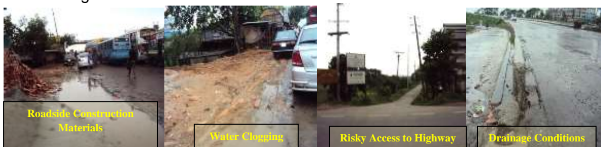
Figure-14: Additional features of the investigated road
